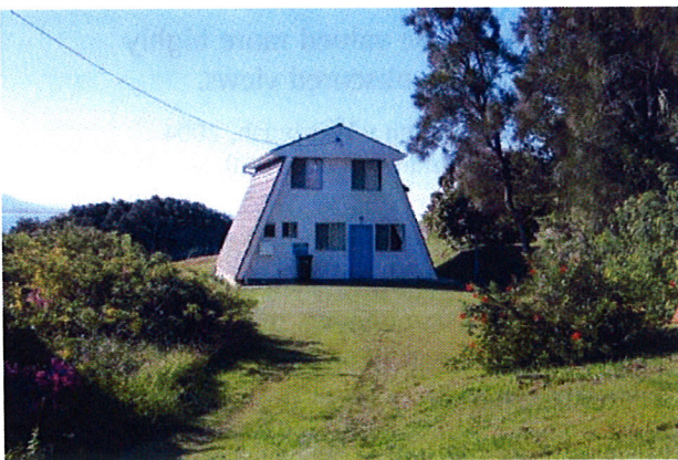
Example of varied building form
